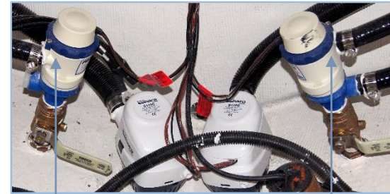
Pumps To Fill Valves
